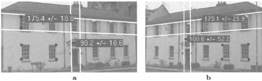
Fig. 4.15. Different views, different computation points. a and b two images of the Crystallography Labs, Oxford. The actual height of all the windows is 174 cm, the door width is 100cm. Notice the correct computation of parallel lines.
