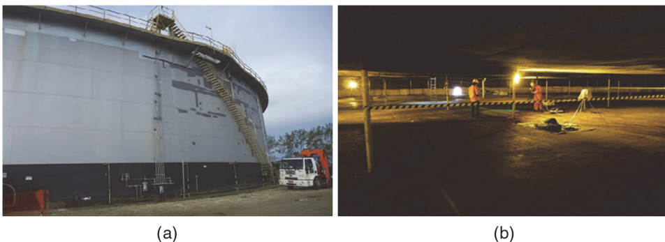
Figure 7.15 (a) External and (b) internal view of a petroleum storage tank (reprinted from Martins de Souza 41 with permission).
