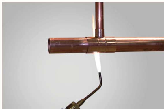
Figure 7.14. Preheating Fitting
