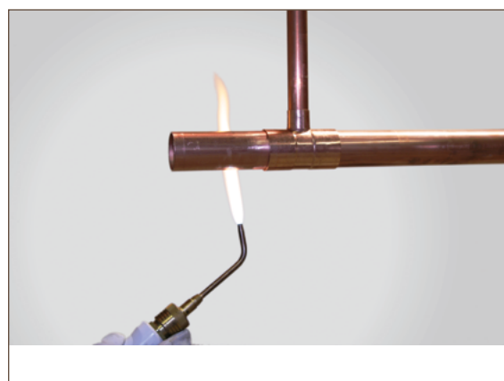
Figure 7.13. Preheating Tube
