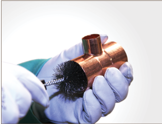
Figure 7.8. Cleaning: Fitting Brush
