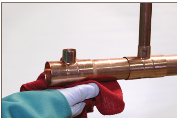
Figure 7.12. Removing Excess Flux
