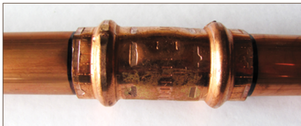
Figure 11.16. Completed installation of a press-connect joint
