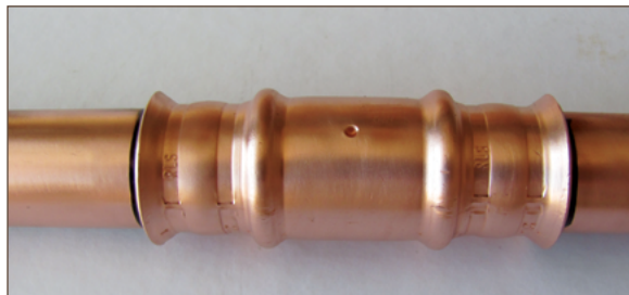
Figure 11.19. Completed joint with insertion marks visible
