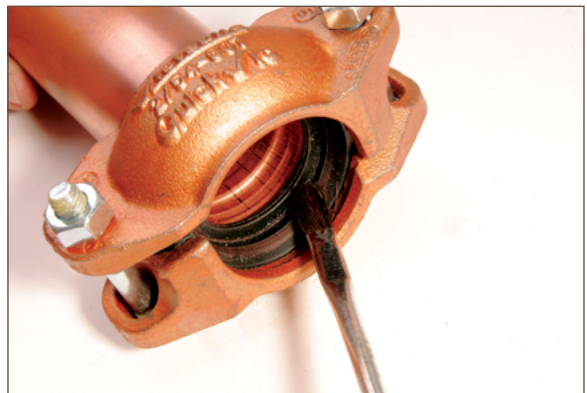
Figure 10.8. Applying lubrication to gasket
