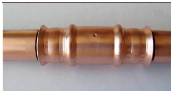
Figure 11.17. Completed joint showing double 360° crimps
