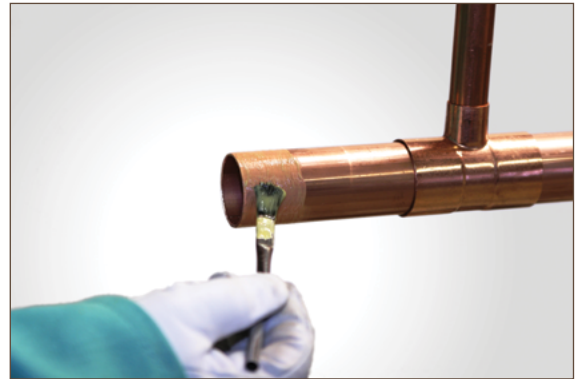
Figure 7.9. Fluxing: Tube
