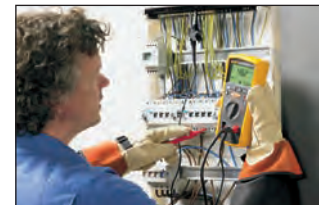
Insulation test at a distribution panel
