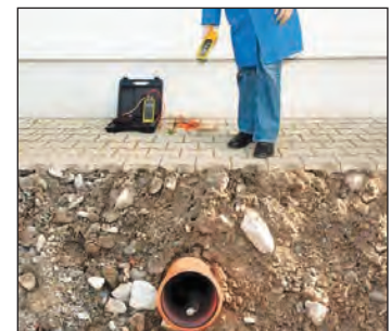
Tracing of underground cables (max. depth 2.5 m)
