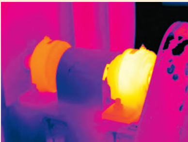
Overheating bearing cap
