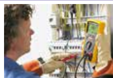
Insulation test at a distribution panel
