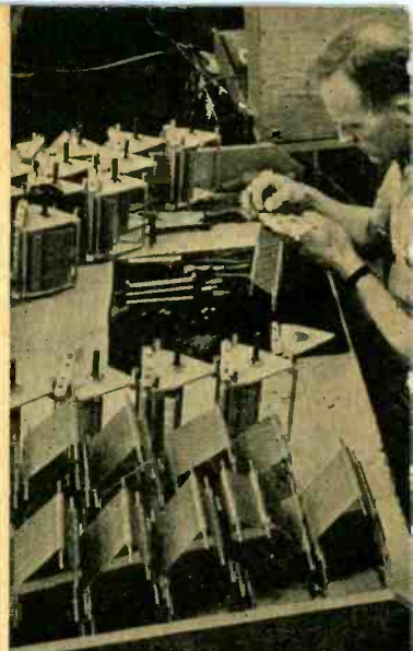
21 - ASSEMBLING OSCILLATOR TUNING CONDENSER
