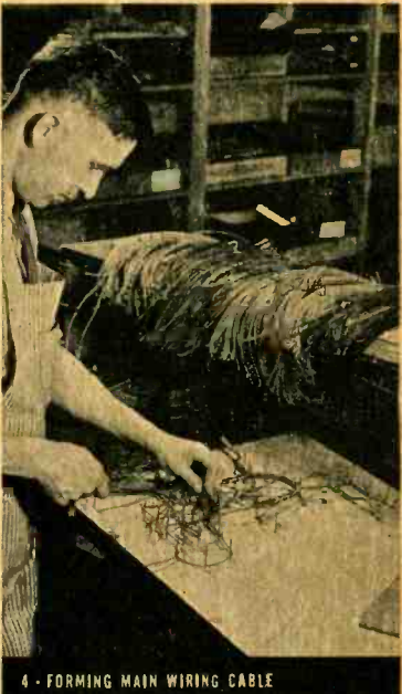
4 - FORMING MAIN WIRING CABLE
