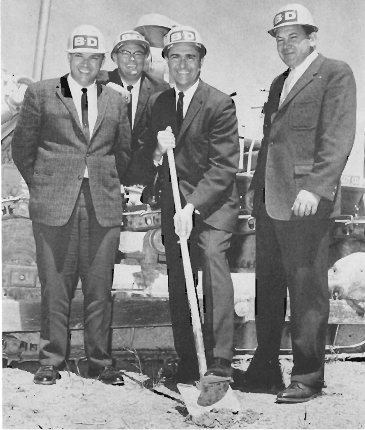
Pete Lahana wields a mean shovel as he officially launches construction of the new Lahana & Company building. Assisting in the ground breaking are (left to right) Marvin King, HP plant engineer at Loveland; Lee Stoner, Lahana field engineer; and A. J. "Mick" Spano, Lahana field engineer.
