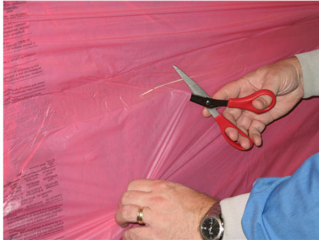
Figure 16: S530 cut the wrap off the system
