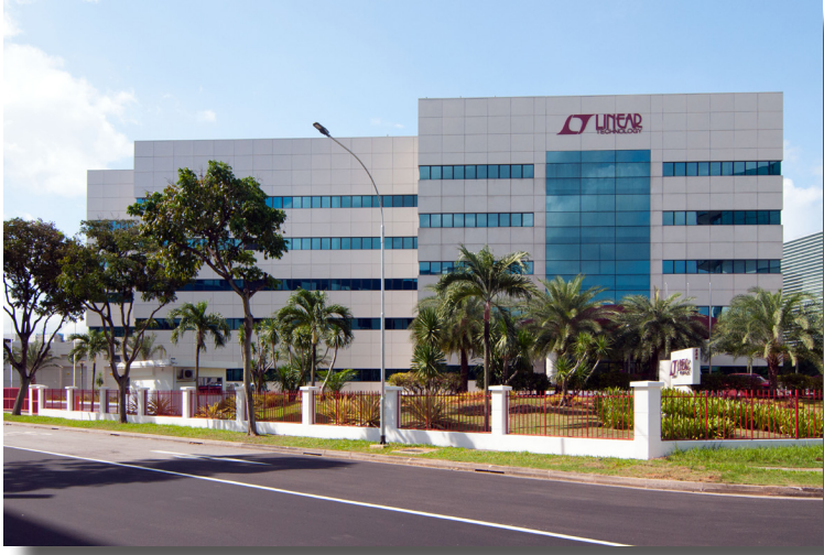
Linear's Singapore test facility expands to boost production capacity.
