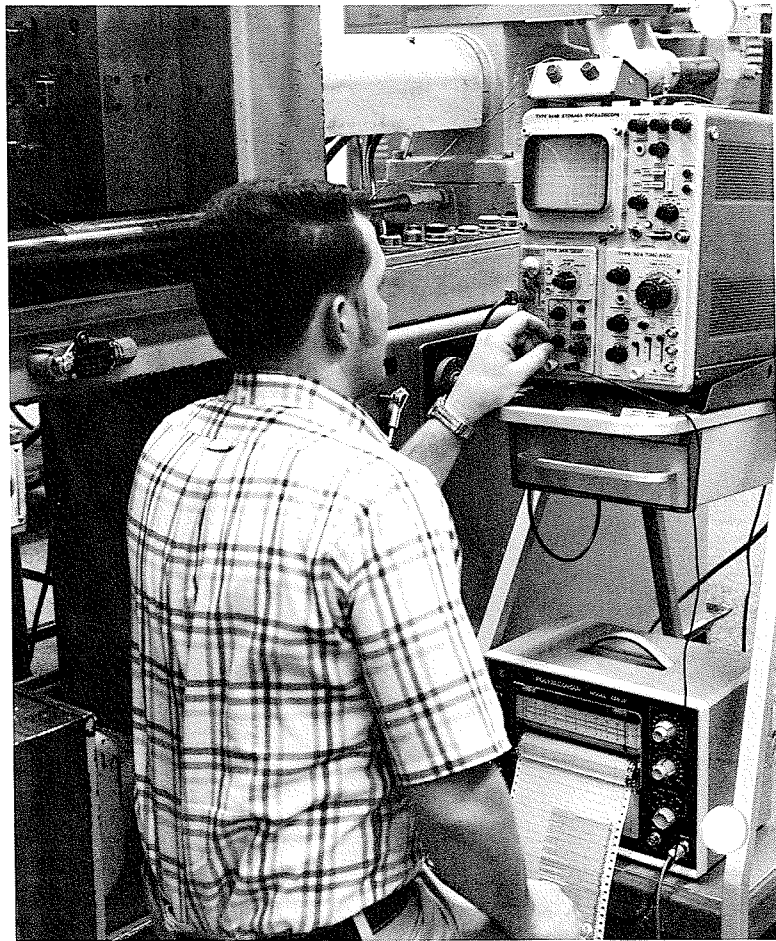
Denny Magden of Plastics adjusts the 3A10 transducer system used in monitoring injection molding of cam switch blanks.
