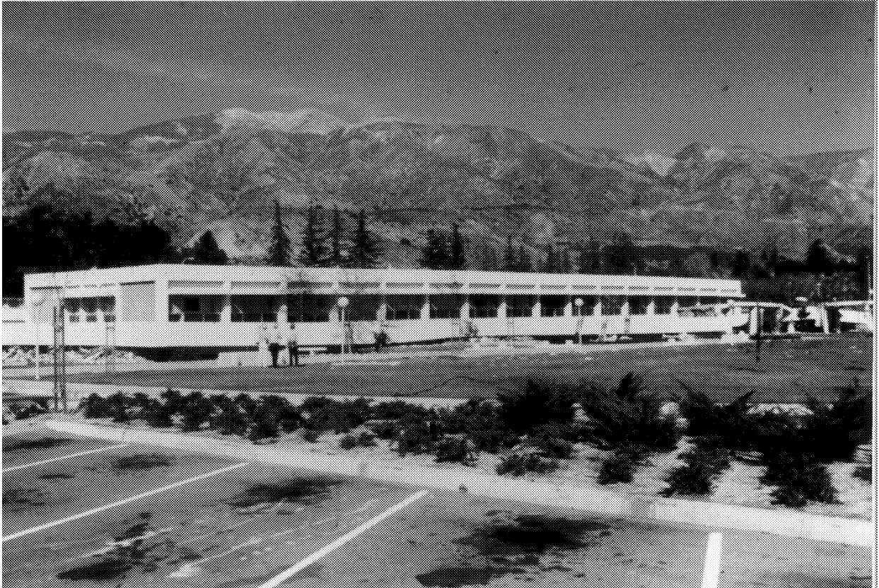
Fig. 1. Collapse of the Psychiatric Unit of the Olive View Medical Hospital (San Fernando Earthquake of February 9, 1971).
