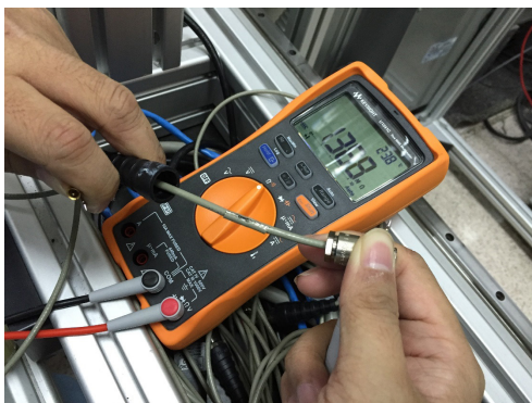
Figure 5: Example of a broken cable close to the connector end
